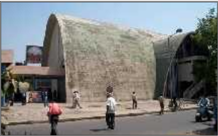
KC THEATRE, SECTOR 17 HAS BEEN DEMOLISHED
