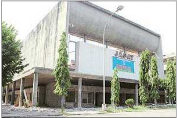
TDI MALL RECONSTRUCTED AFTER DEMOLISHING JAGAT CINEMA
