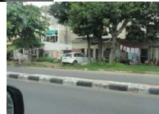
HOUSES WITH DOORS OPENING ON V2/V3 ROADS
