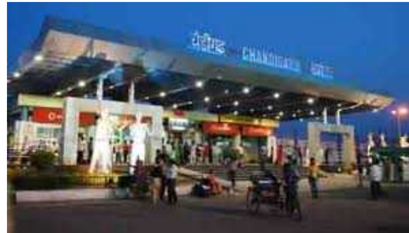
CHANDIGARH RAILWAY STATION
