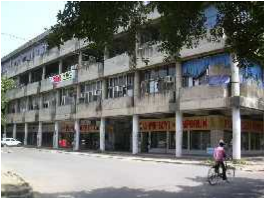
UNAUTHORISED COVERAGE OF COMPULSORY VERANDAH
