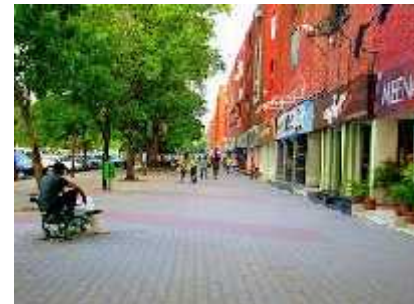
THREE STOREYED ARCHITECTURAL CONTROLLED BRICK BUILDINGS
