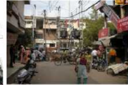
HANGING WIRES-TRANSFORMERS ON MAIN STREETS
