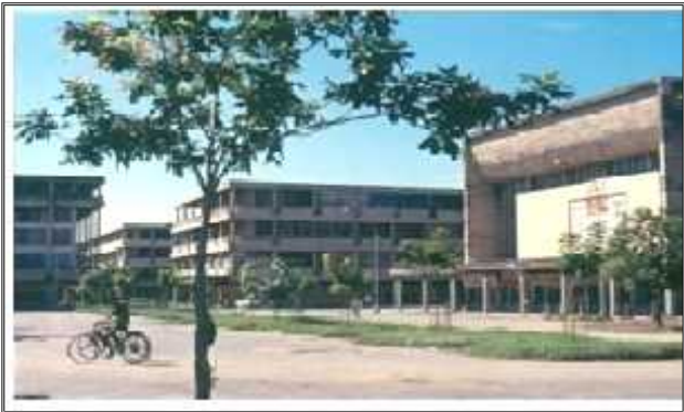
THE JAGAT THEATRE, SECTOR 17 HAS BEEN DEMOLISHED AND REBUILT
