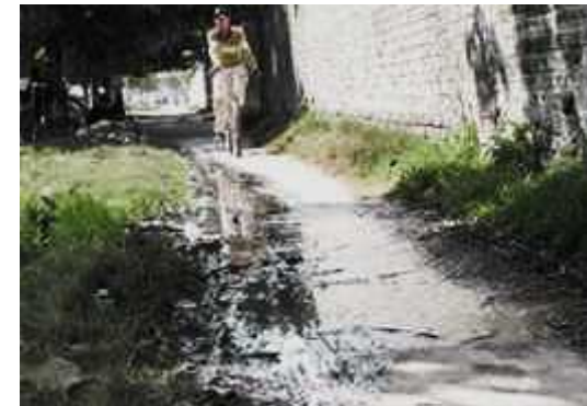
POOR CONDITION OF ROADS AND CYCLE TRACKS
