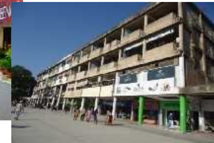
FOUR STOREYED RCC BUILDING
