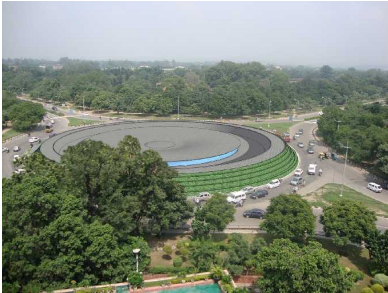
Conceptual Sketch prepared by the Department of Urban Planning, UT, Chandigarh based on DMRC report and details
