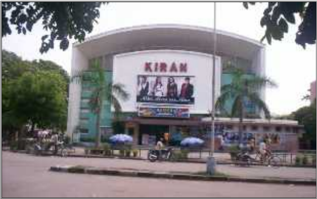
KIRAN CINEMA – RECOMMENDED FOR HERITAGE STATUS
