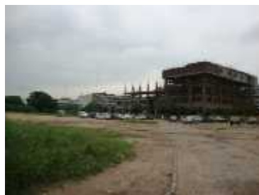
LIBRARY & BLOCK (UNDER CONSTRUCTION VIEW FROM PLAZA)
