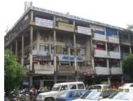
VISUAL POLLUTION DUE TO SIGNAGE, BLACKENING AND WEATHERING OF FACADES ACUTE SHORTAGE OF PARKING
