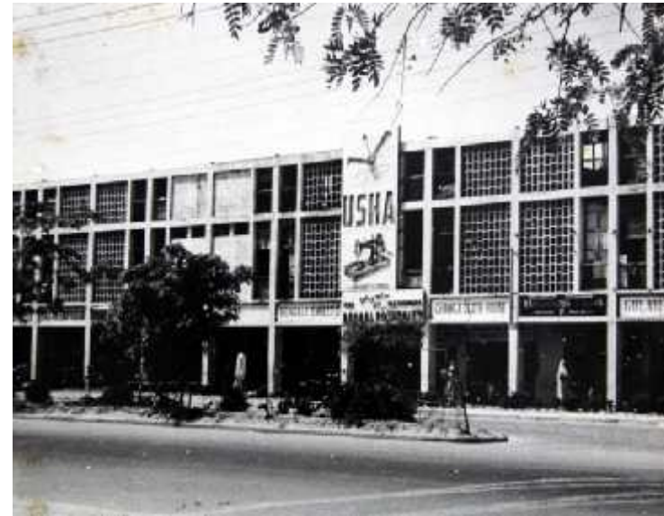
ORDERLY ORIGINAL FACADES OF THE SHOPPING CENTRES, THROUGH SIGNS OF VIOLATIONS HAD BEGUN TO SURFACE
