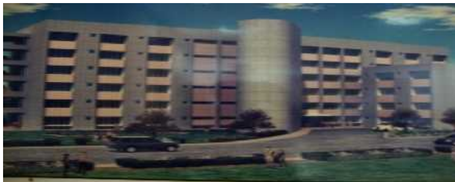
3D VIEW OF THE NEW OPD BLOCK OF THE MULTI SPECIALTY HOSPITAL, SECTOR 16
