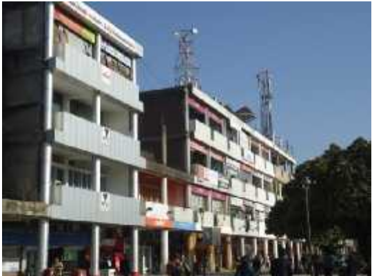
PAINTING/ PLASTERING OF FACADE & COLUMNS
