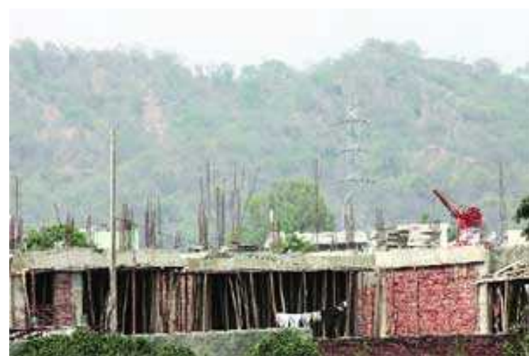
Construction of School and village Kaimbwala
