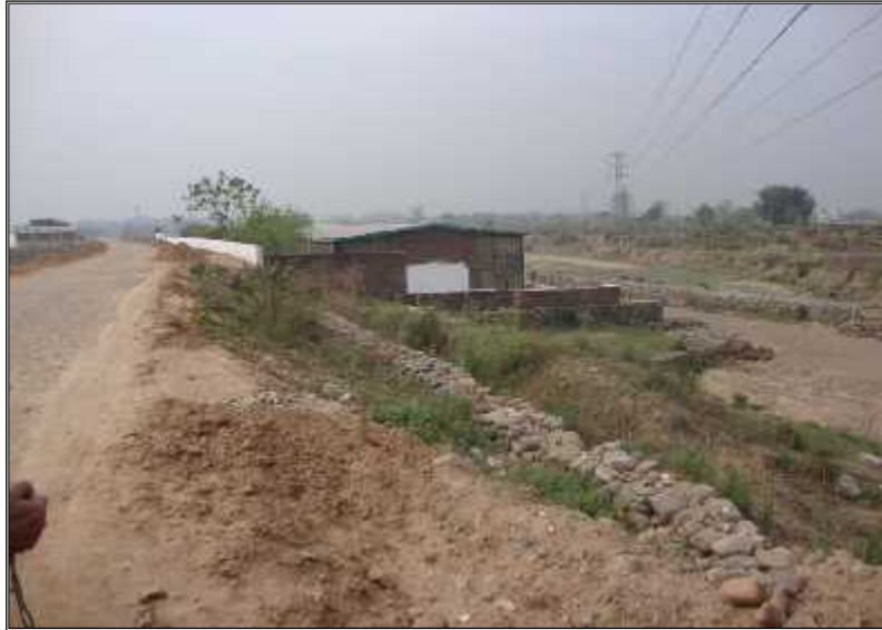
ENCROACHMENTS WITHIN THE NATURAL RIVULETS
