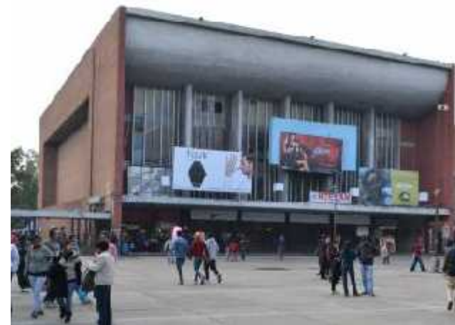
NEELAM THEATRE – RESTRUCTURING OF THE THEATRE IS IN THE OFFERING (CONSTRUCTION YET TO BE INITIATED)
