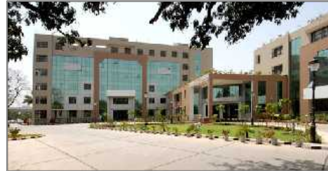
NEWLY CONSTRUCTED HARYANA OFFICE BUILDING, SECTOR 33
