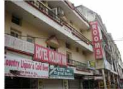
COMMERCIAL ACTIVITY SPREAD ACROSS FLOORS
