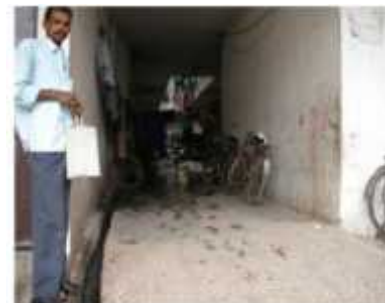
NARROW APPROACH AND INDEQUATE SOURCE OF LIGHT
