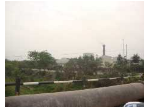
Dumping ground -garbage treatment plant along Patiali-ki-Rao, Dadumajra. The city's garbage disposal sites are located towards the, western periphery of the city. The residents resent the air pollution and smell generated .
