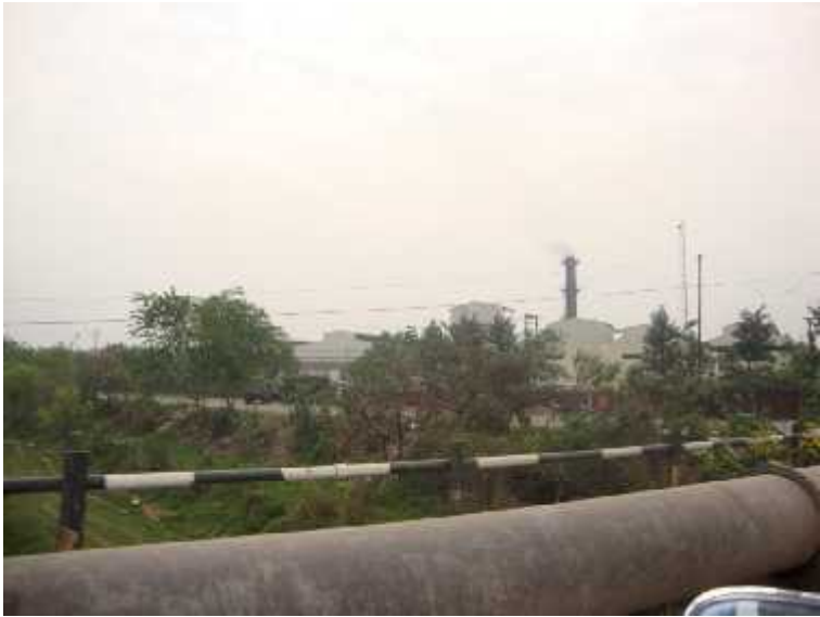
GARBAGE TREATMENT PLANT ALONG PATIALI-KI-RAO, DADUMAJRA
