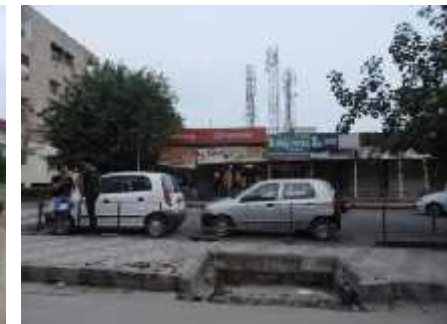
POORLY MAINTAINED UTILITIES.
