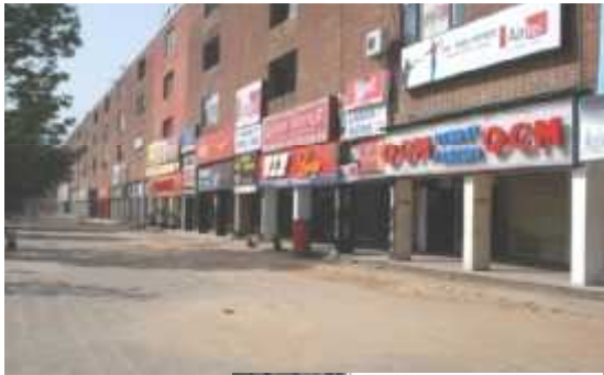
VIOLATION OF ADVERTISEMENT CONTROL
