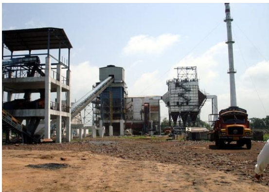
Biomass Gasifier Installed at, Vill Banki, Block Bodla, Dist. Kawardha
