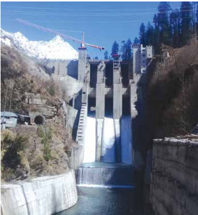
PARBATI STAGE-II, HIMACHAL PRADESH
