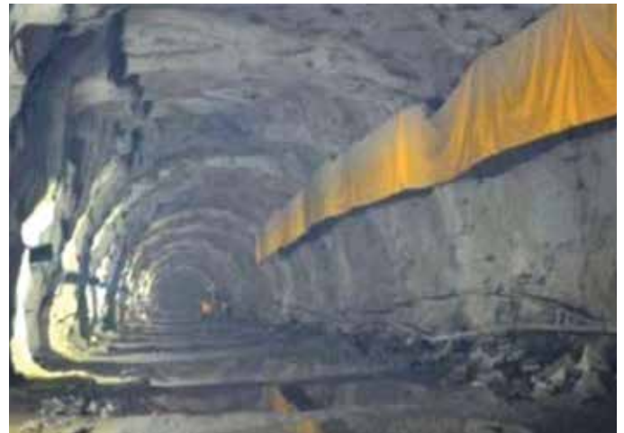
Luhri Stage-1 HEP (210 MW) - Diversion Tunnel Construction
