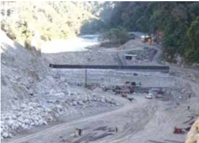
Arun-3 HEP (900 MW) - Cofferdam Area Construct
