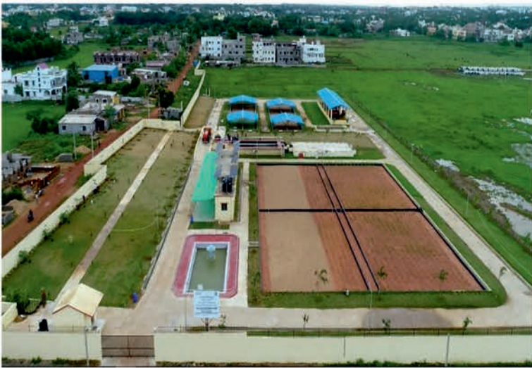
Septitized treatment plant at Bankabija, Basuaghai, Khordha
