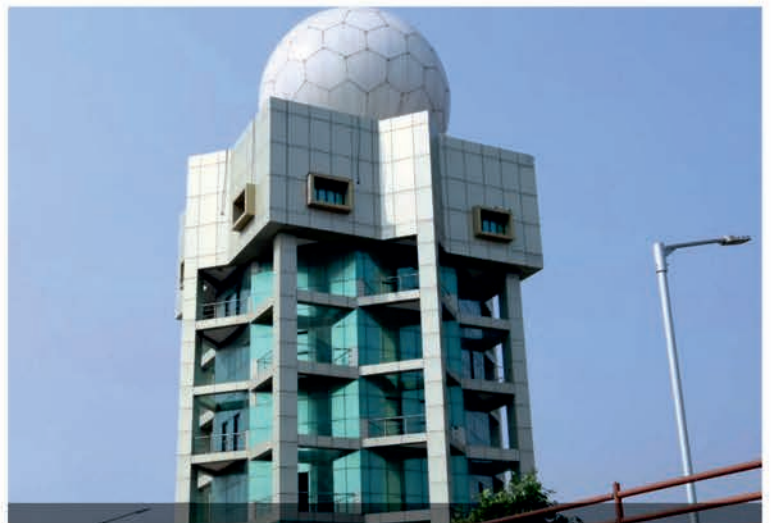
Doppler radar installed at Paradeep
