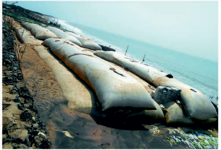
Geo-Synthetic Tube Installation at Pentha, Kendrapada
