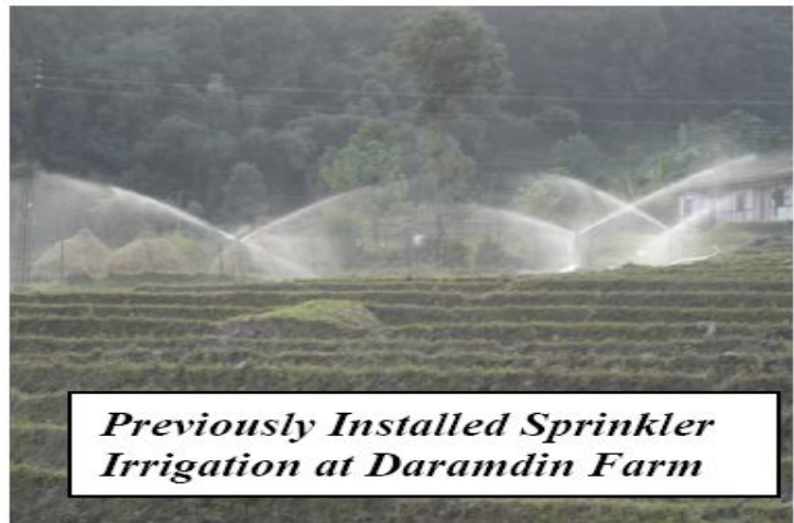
Figure 7.4a: Sprinklers being used
