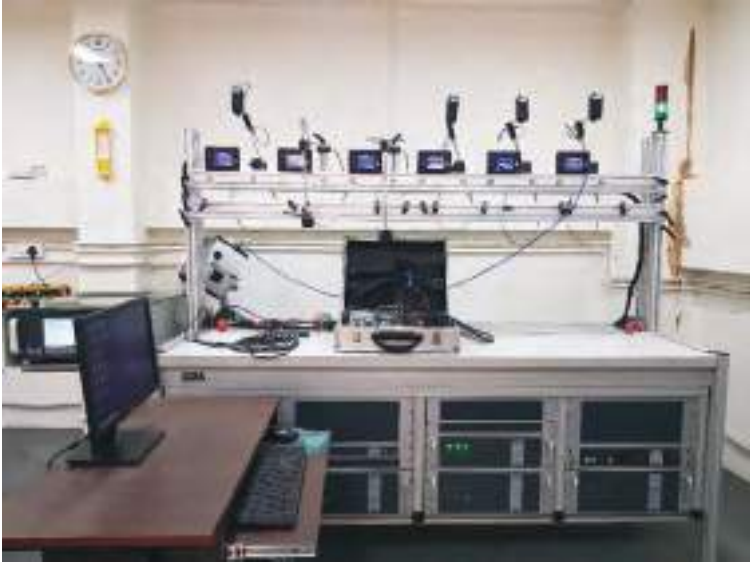
High Precision Automatic Smart Electric Meter Test Bench procured, installed and commissioned during 2021.
